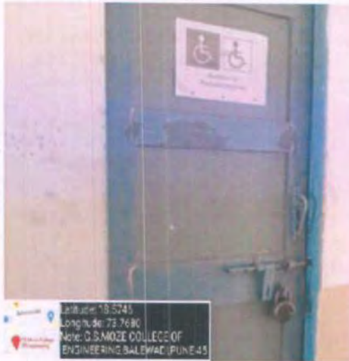
Restrooms on ground floor
