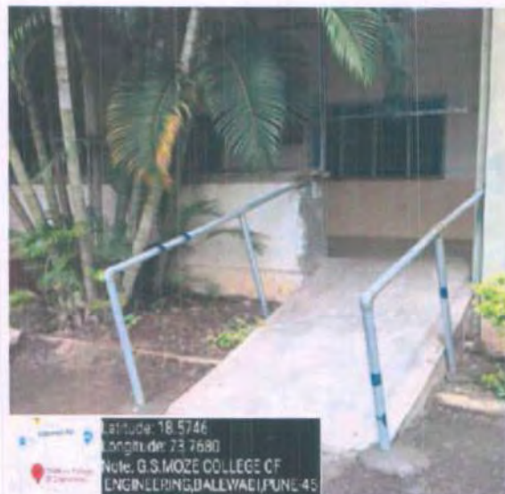
Ramp for classrooms and labs
